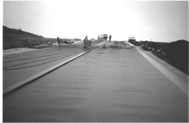
Figure 5. Example of a flat geomembrane on a landfill slope.
